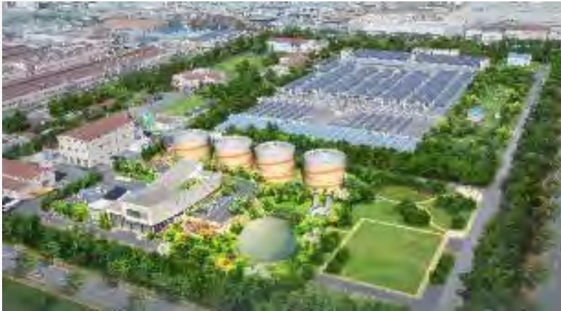
Noksan WWTP in Korea - Side-Stream AMX (780 ton/day)
