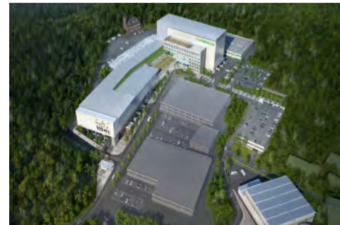
Pukyong Nonghyup Organic Waste Treatment
