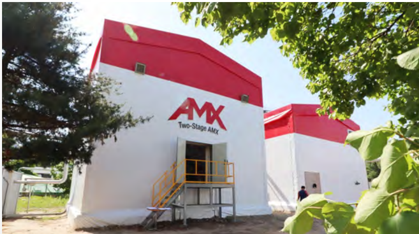
Daejeon WWTP - AMX Incubating facility (220 ton/day)
