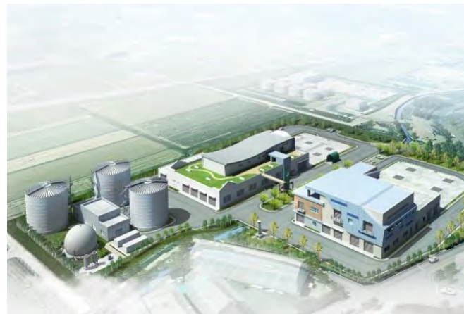
Gimhae Livestock Wastewater Treatment Plant
